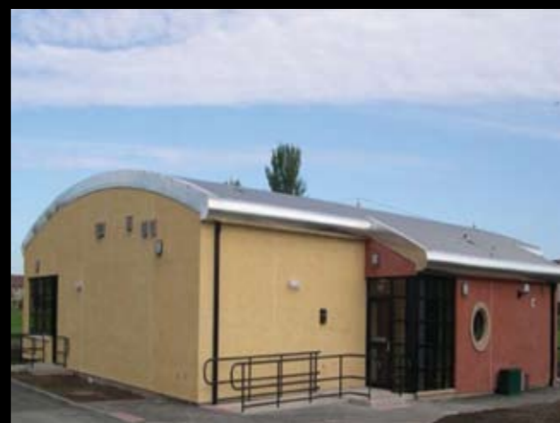
Base coat 10-12mm Dash receiver 4-6mm Roughcast
