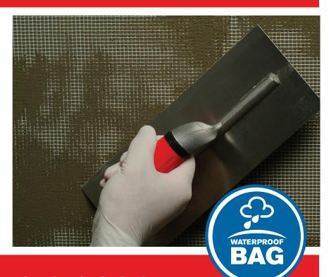
RapidMix Base Coat Render is a cement-based render that has been modified in order to offer improved adhesion, water resistance and workability.
