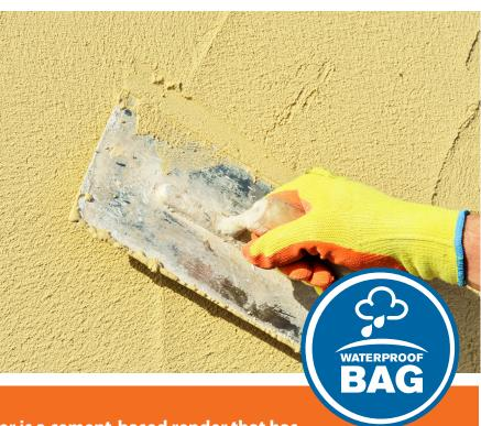
Rapid Mix Multi Finish Coloured Render is a cement-based render that has been modified in order to offer improved adhesion, water resistance and workability.
